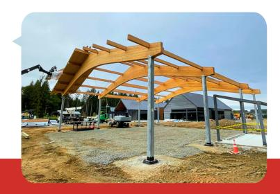
The Black Diamond Pickleball Court boasts four Large Peak and Camber Glulam Beams, each playing a crucial role in the structural integrity and visual impact of the shelter.
