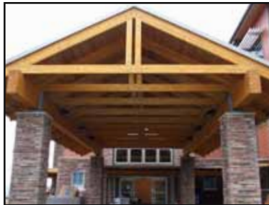
Medical Office Building in Issaquah, WA
