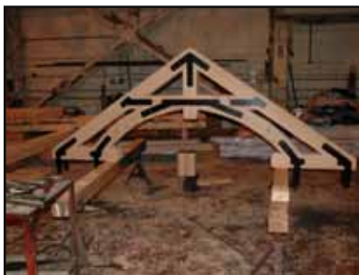
Residence truss during fabrication in our shop
