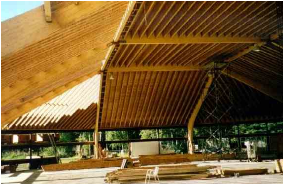
Figure 4. Birchwood Community Church in Anchorage, Alaska. These glulam arches were sized to achieve a one-hour rating. The roof-ceiling assembly will have two layers of 5/8" (16mm) gypsum wallboard attached to the bottom of the roof joists. The steel connections will be covered with 2x wood blocking.
