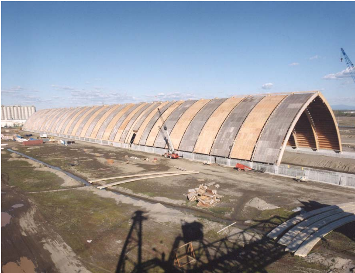
Figure 1A. This 1476 ft (450m) building is used to store potash, a chemical used in fertilizer. The glulam arches span 161 ft (49m) and are spaced at 32 ft (9.75m) on center. The glulam purlins are 3 1/8" x 16 1/2" (79mm x 419mm) and are spaced at 48" (1219mm) on center. The roof sheathing is 1 1/8" (28.6mm) thick plywood. This building classifies as Heavy Timber Construction.
