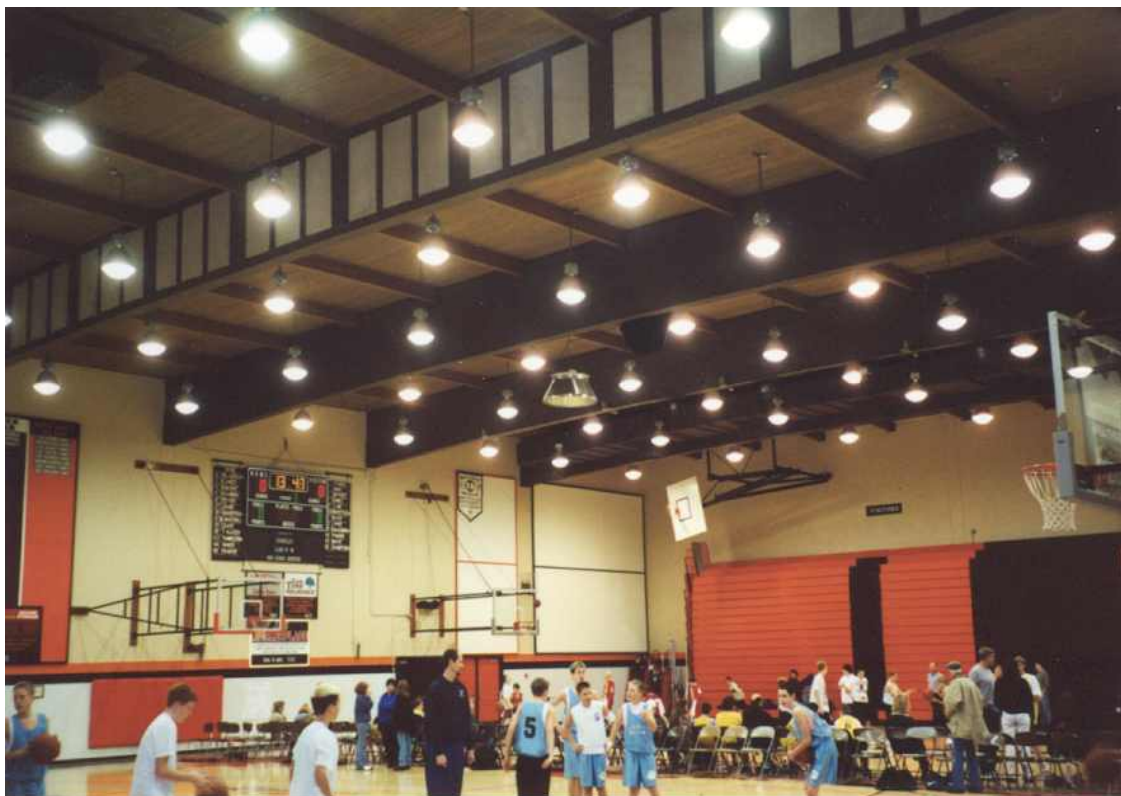
Figure 1. High school gymnasium with heavy timber roof. Notice the large main and secondary beams and 2 x 6 tongue and groove decking.
