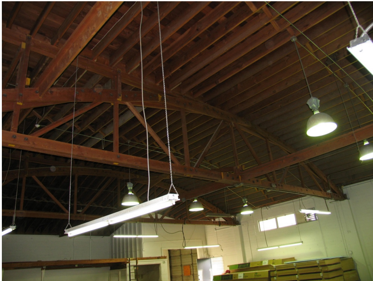
Photo #7. Truss with over-framing on one side.
