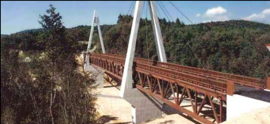
At 16' x 475', this award-winning, cable-stayed bridge in Japan is the longest clear-span timber vehicular bridge in the world.
