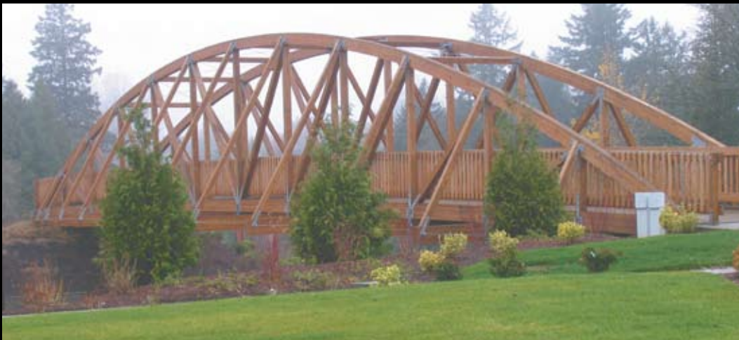
A 10' x 136' bowstring truss pedestrian bridge, assembled on-site and installed using a crane.
