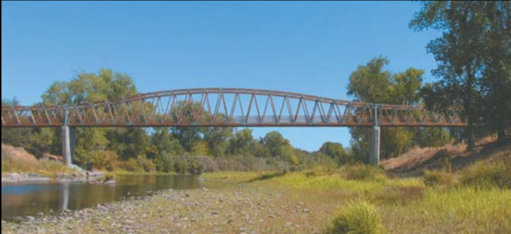
One of the longest timber bridge spans in the United States, this structure in California measures 12' x 410'.
