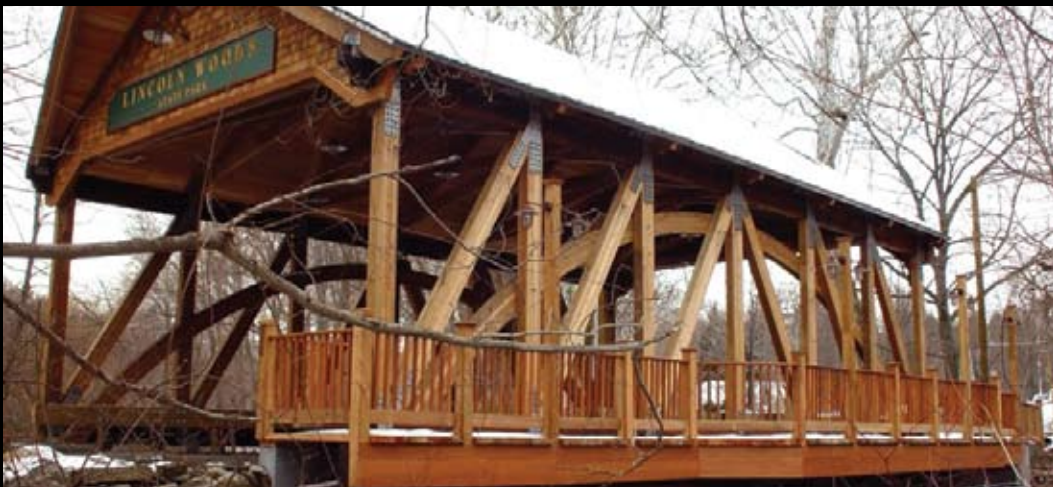
This modern day example of a covered bridge in Rhode Island offers an adjacent fishing pier. A decorative arch was used to enhance aesthetics.
