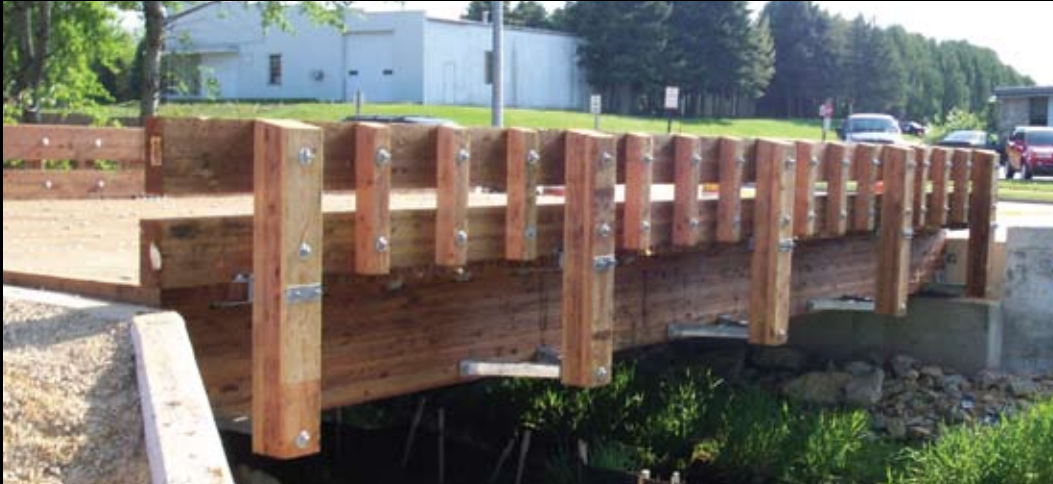
This 24' x 36' vehicular girder bridge is designed to carry a load of 72,000 lbs (HS-20), and includes a decorative rail.
