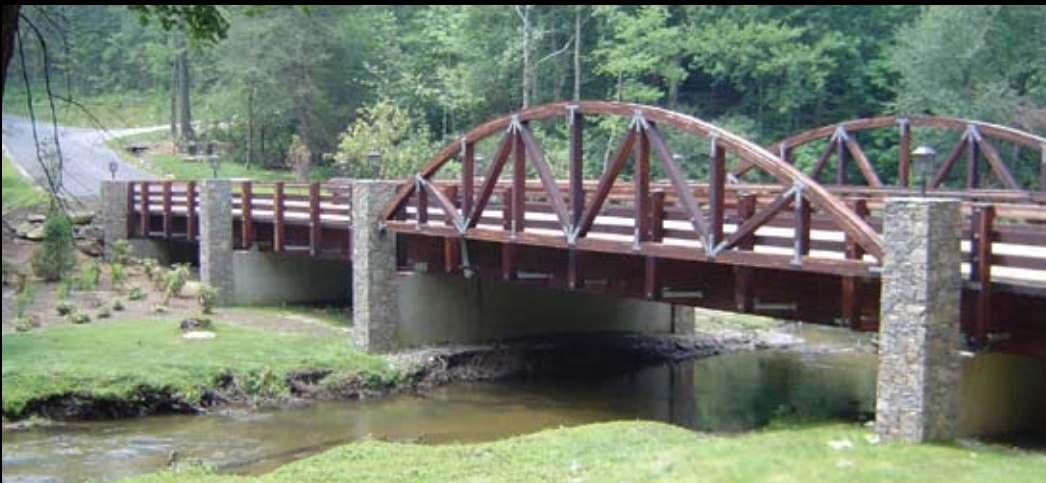
28' x 150' four-span, vehicular girder bridge with simulated bowstring truss in North Carolina.
