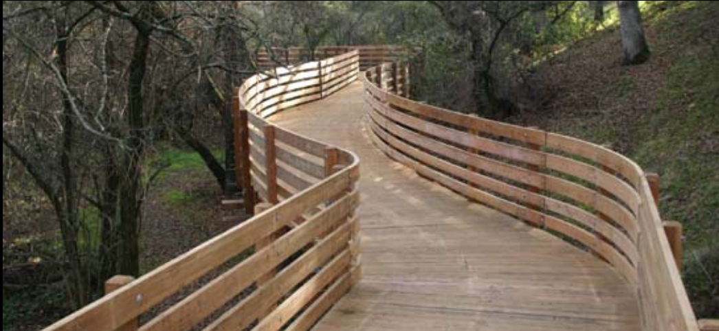
This 180' pedestrian bridge in California includes two 60-ft. clear span sections, and employs a radiused rail system in order to minimize environmental impact.
