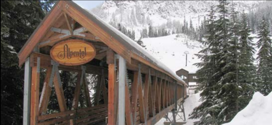
A 10' x 285' parallel chord truss covered bridge with a roof designed to withstand a 430 psf snow load.
