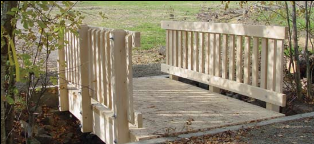
This 6' x 11' pedestrian bridge requires no preservative treatment since Port Orford Cedar is a decay-resistant species.
