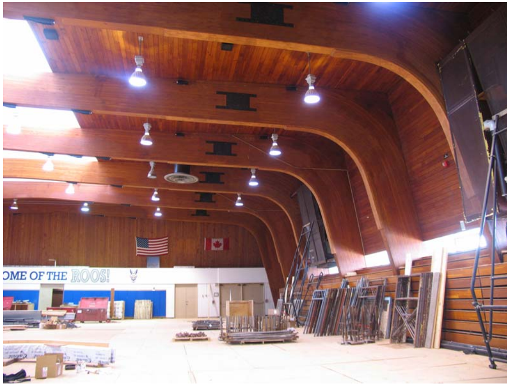
Figure 14. Frames with structural repairs complete, sanded and stained.
