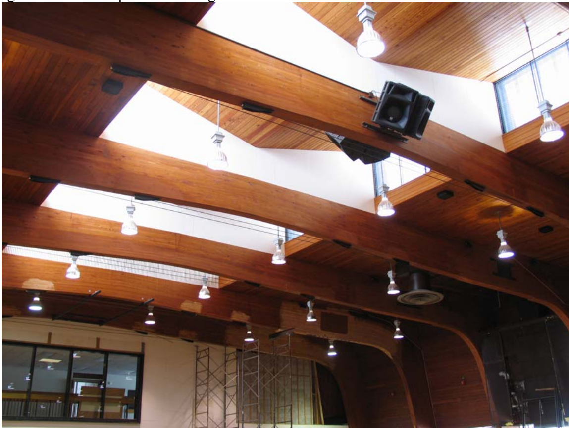
Figure 8. Post tensioning cables attached to beam soffit.
